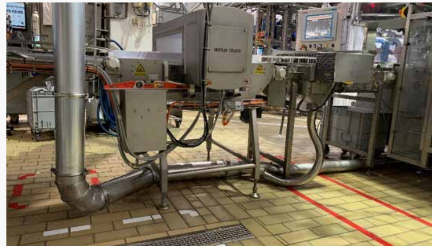
The individual conveying lines from each production machine make it possible to keep different waste materials/colours separated.
