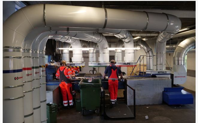
Suction points at the sorting line reduce repetitive lifting, twisting, and throwing.
