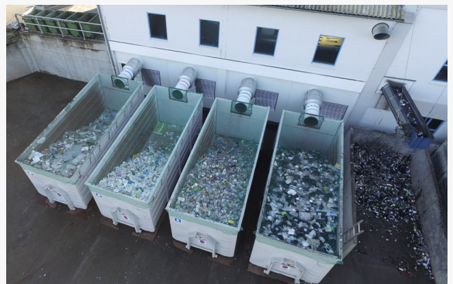
Separated material streams are conveyed directly to outdoor collection containers.
