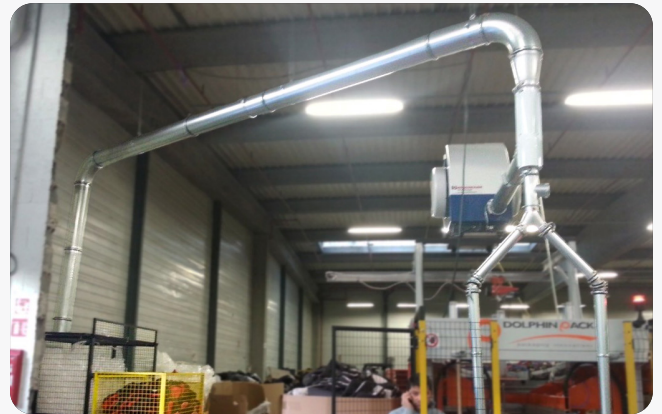
The pneumatic solution secures efficient handling of the plastic trim from all eight conveying lines.
