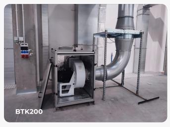
**The BTK blower** is designed for continuous transport of materials, like shredded film scraps, through a closed loop conveying system.
