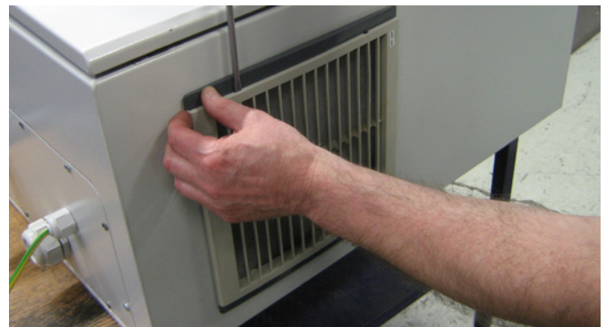
1 - press both clips to release the plastic frame.
