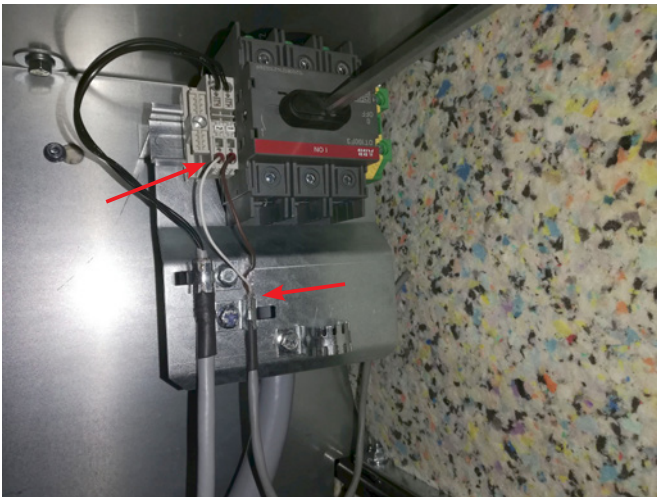
3 - The wires for the ptc sensors are routed as shown, and connected in the terminal block. Also secure the wires with the cable relief, ensuring shield braid contact.
