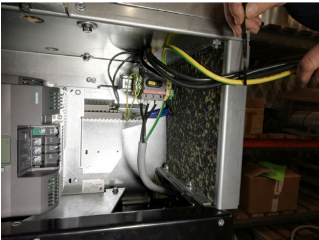
27 - and secure the cables with a cable tie as shown, away from the AC drive
