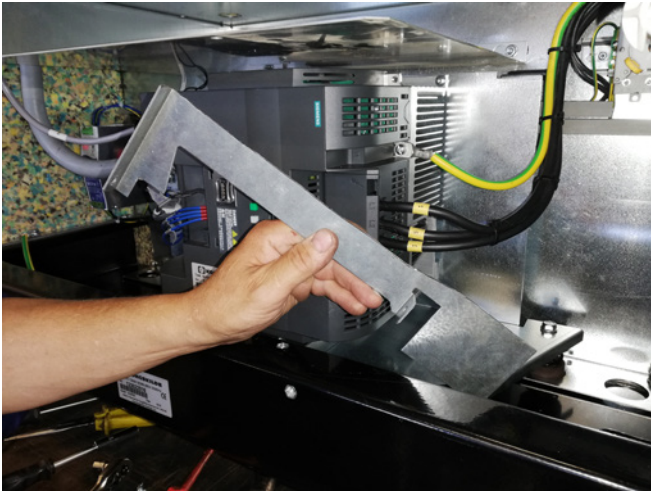
37 - refit the vertical bracket, and tighten the screws
