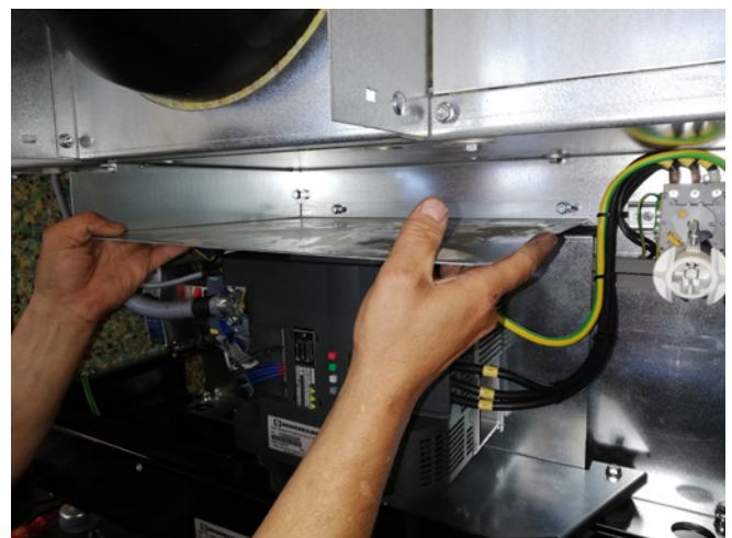
36 - refit the horizontal bracket, and tighten the screws
