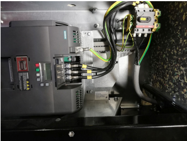
26 - remove the contact screws for the supply cables from the main switch
