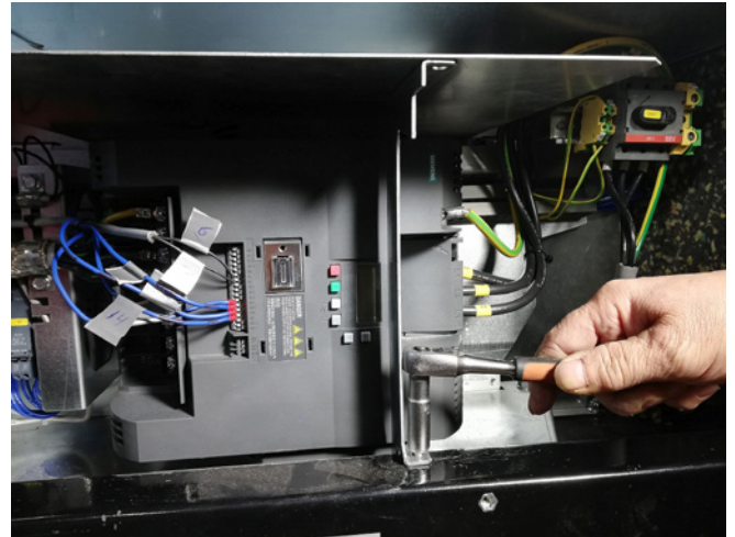
22 - loosen the vertical bracket by removing 2 screws , 1 in top and 1 at bottom, and pull out the bracket
