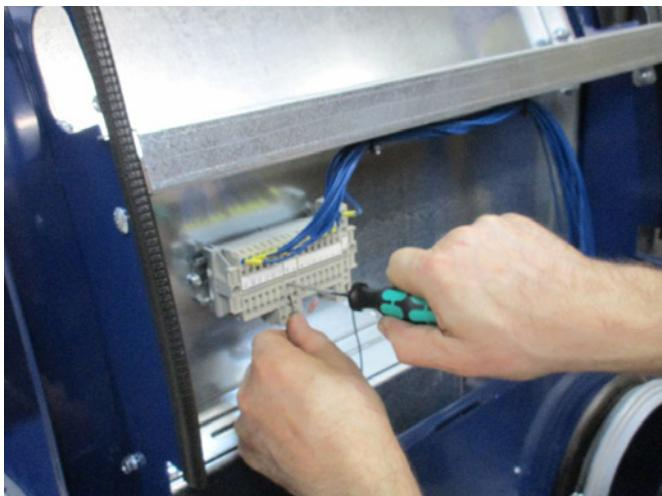
4 - The cable relief is tightened and the blower cover refitted.
