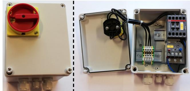
The external motor control is connected in terminal block X30 between terminal 2 (0 VDC) and 16 (Digital Output 3) and a loop is installed between terminal 1 (+24 VDC) and 12.
