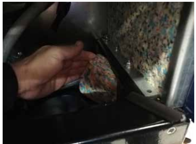
4 - insert the enclosed four foam blocks in both left and right side of the blowers bottom frame, and push the blocks forward / sideways, as far as possible. These blocks will close the metal sheet gaps in the bottom frame.
