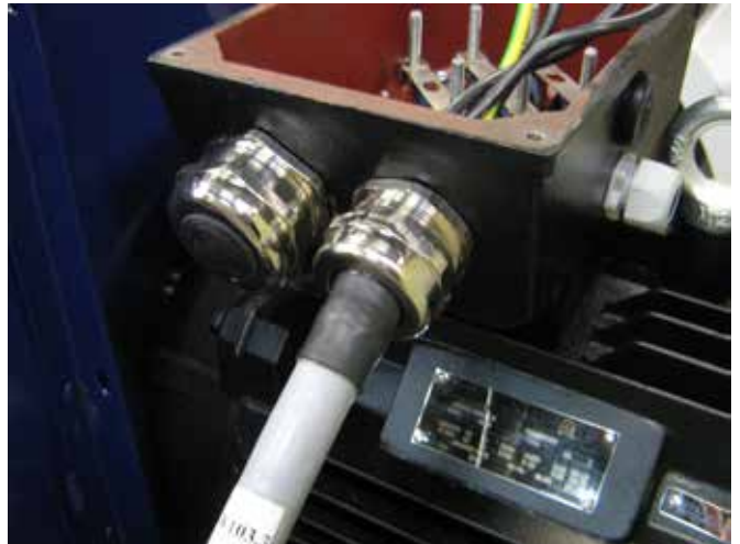
7 - make sure the cable is seated as shown.
