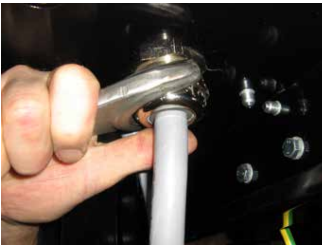
10 - tighten the cable relief for power supply and thermostat cables.
