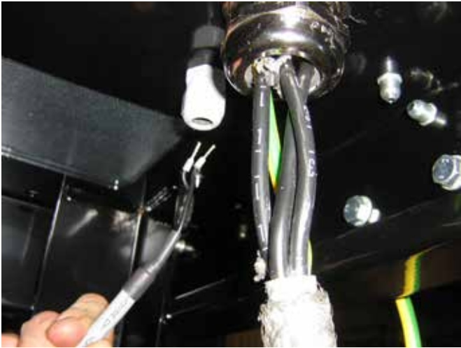
3 - the cable relief unions are loosened. The power supply and thermistor cables are guided through the bottom plate of the blower.
