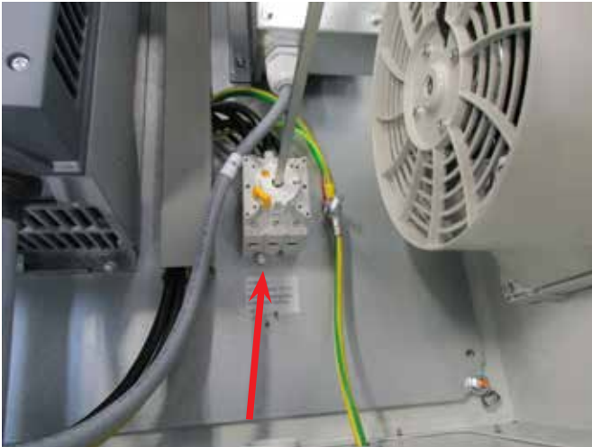
15 - power supply cable is connected to the main switch as indicated.
