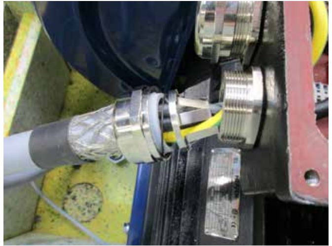
6 - the power supply cable is guided through the cable relief, and the relief ring installed as shown.
