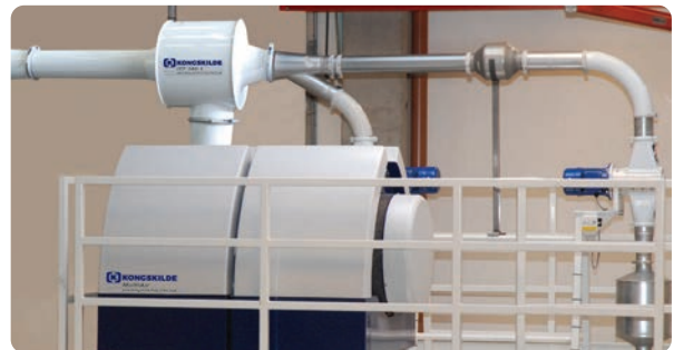
| ITF venturi powered by a MultiAir blower.
