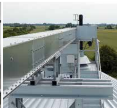
Motor rain cover for outdoor installation.
