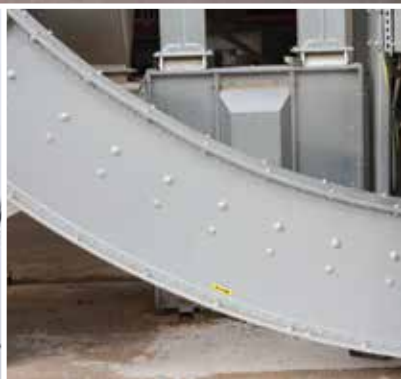
45° angle bend for KCA chain conveyor.
