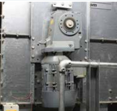
Compact drive solution with bevel gear motor.
