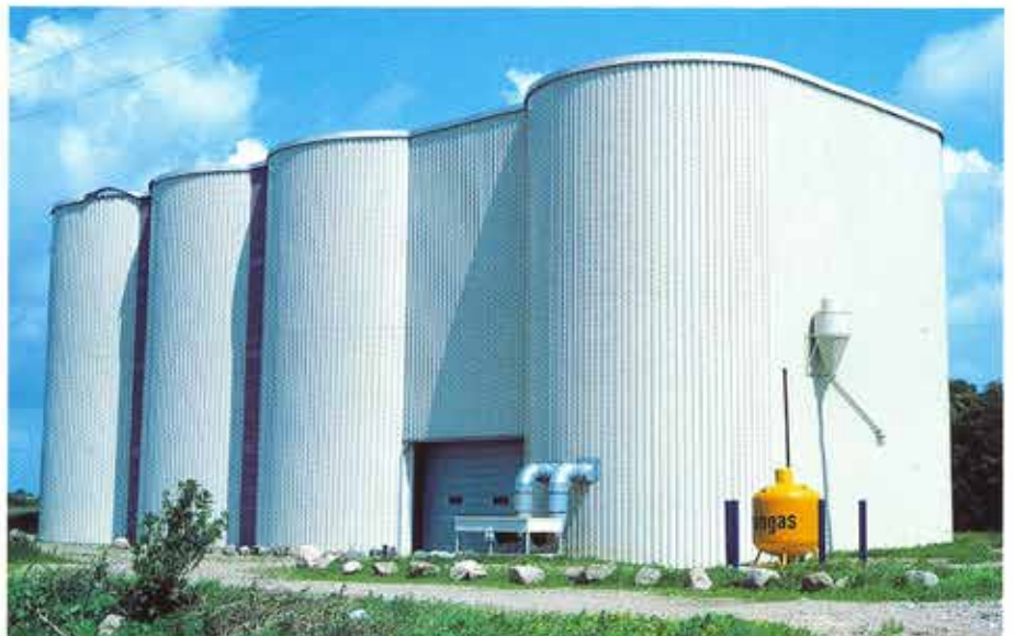
1800 ton grain drying and storage silo, Denmark.
